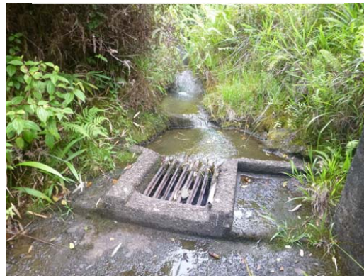
Kolea Stream Intake on Wailoa Ditch
